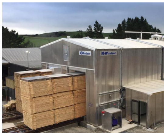
Figure 7: Geothermal-Kiln drying timber 28 .
