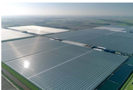
Figure 5 Hoogweg Paprikakwekerijen greenhouse operations spanning 160 hectares (www.hoogweg.nl)
